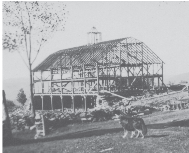
Lawrence barn frame is finished. Note the gambrel roof style.
