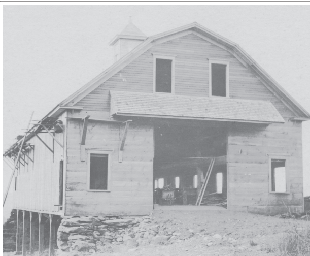
The barn frame is closed in and the top portion is clapboarded. Note the pent roof over the main door.
